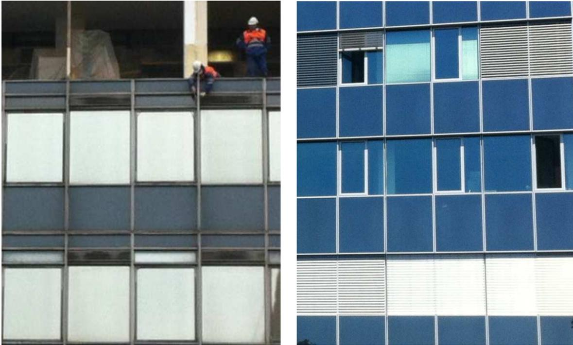
**Figure 1 - left: the original curtain wall during disassembly (March 2013), right: the new curtain wall (July 2013). In both cases we can observe indoor and outdoor venetian blinds and different window openings.**
